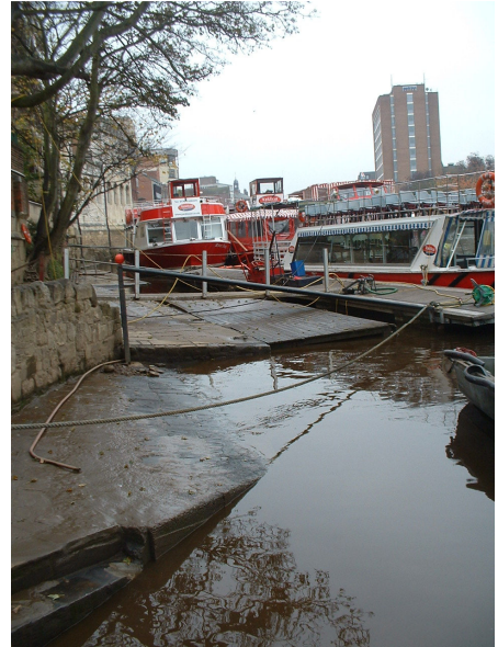
Lendal Boatyard where scouring by the river has created need for repairs
